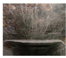
A crack like this can allow deadly gases to leak into the home, and can open the way for a chimney fire to turn into a house fire
